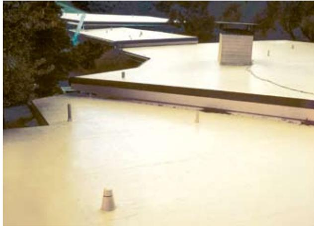
3-inch insulated foam. Finally, a decorative redwood trim was added around the edge. It was painted, along with all of the metal on the roof, to match the tan membrane.
