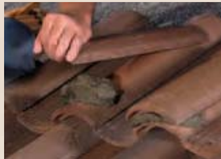
Placing The Mortar
