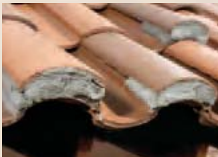
Close-Up of Boosted Eave
